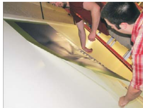
Peel release liner evenly as graphic is applied.
