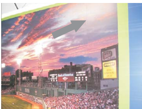
Once panels are complete trim with a sharp utility knife overlap to eliminate bump
