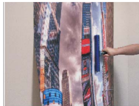
Use the roller working from the center out to apply graphic. If a spot is uneven simply pull from wall or substrate and re-apply. SyntiSOL will not stretch like vinyl
