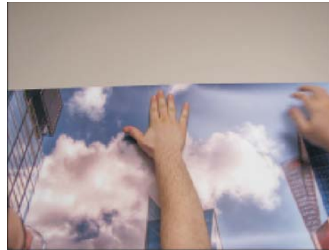
Place image in desired location. Always apply from center out
