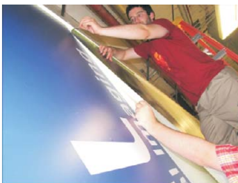
For the next panel use string and edge of previous panel. SyntiSOL 3529 is forgiving to apply and re-apply for correct position.
