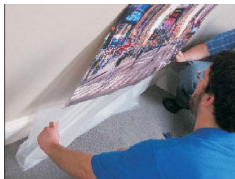
Remove final portion of release liner and apply from center out
