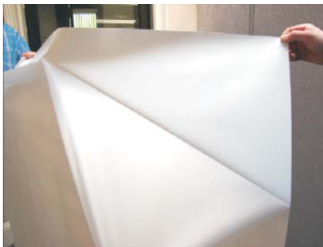
Peel back a few inches of release liner to create a hinge.
