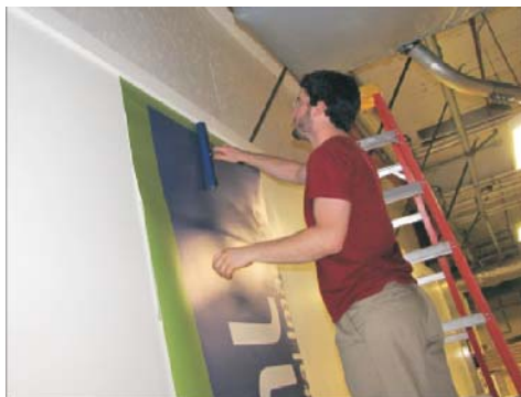
Position image and use the roller to press from the center out.
